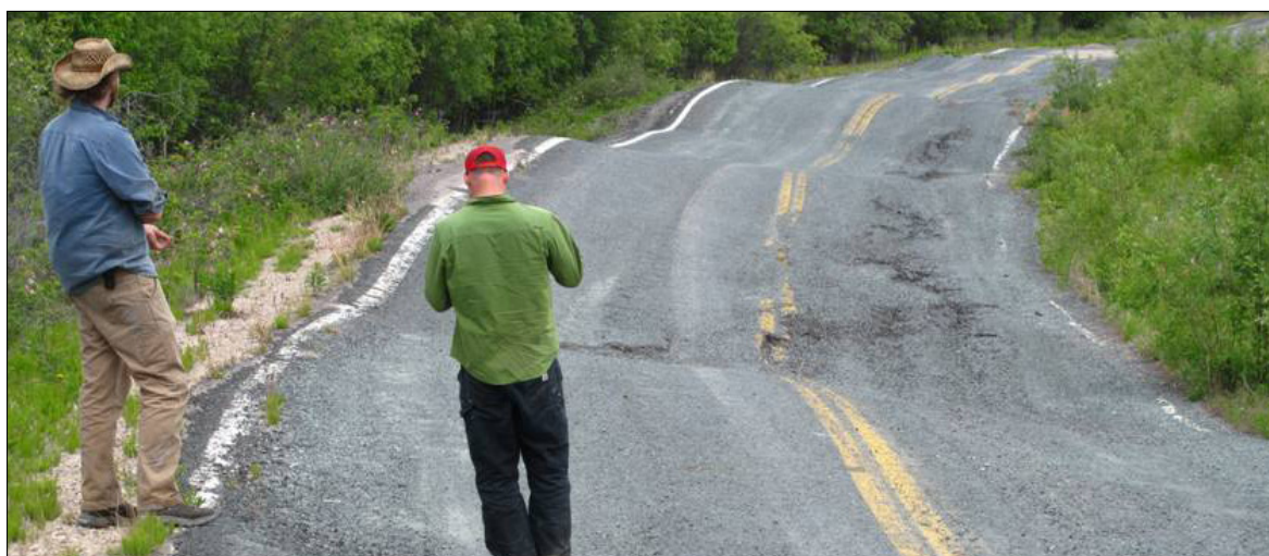
Figure II.2.1 Differential settlement associated with permafrost thaw along an abandoned section of Northwest Territory Highway 4, east of Yellowknife
