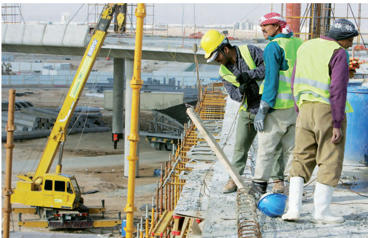
Construction workers, Gulf Region
