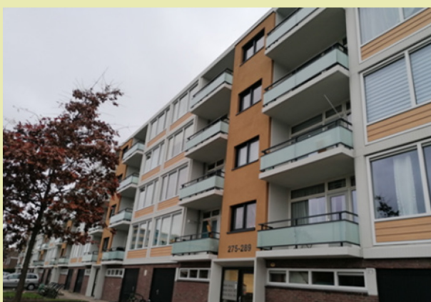
Retrofitted building in Utrecht.
