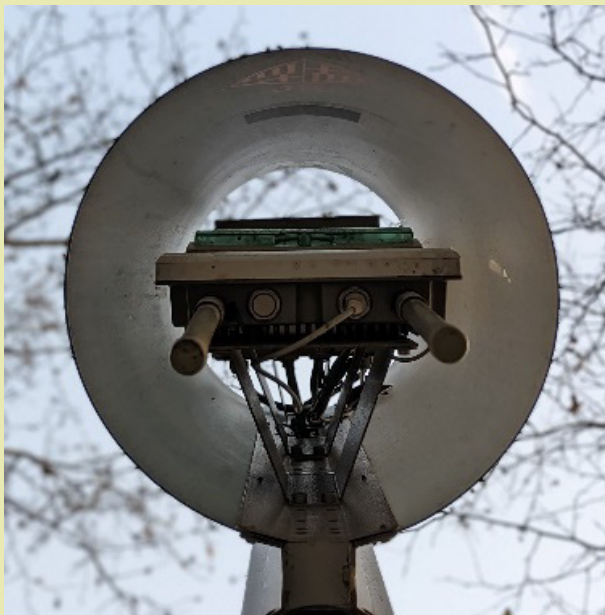
Smart tower in Barcelona.
