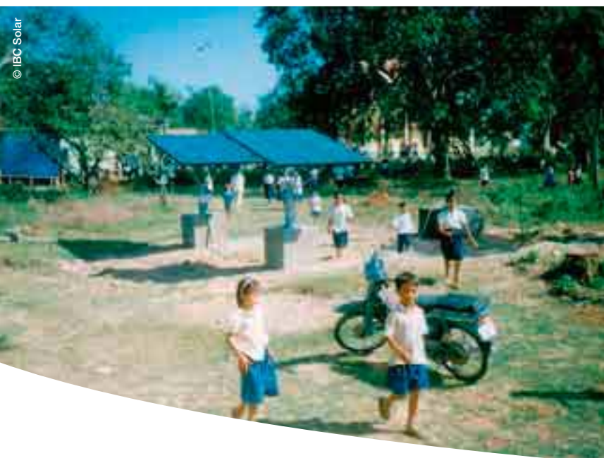
PV system in a school in Cambodia
