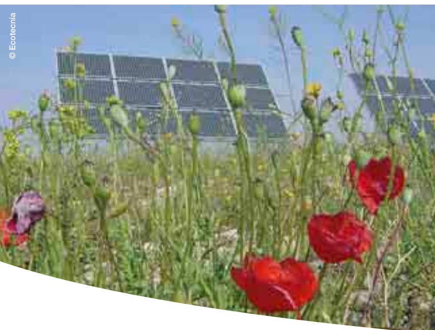
Large solar power plant in Spain
