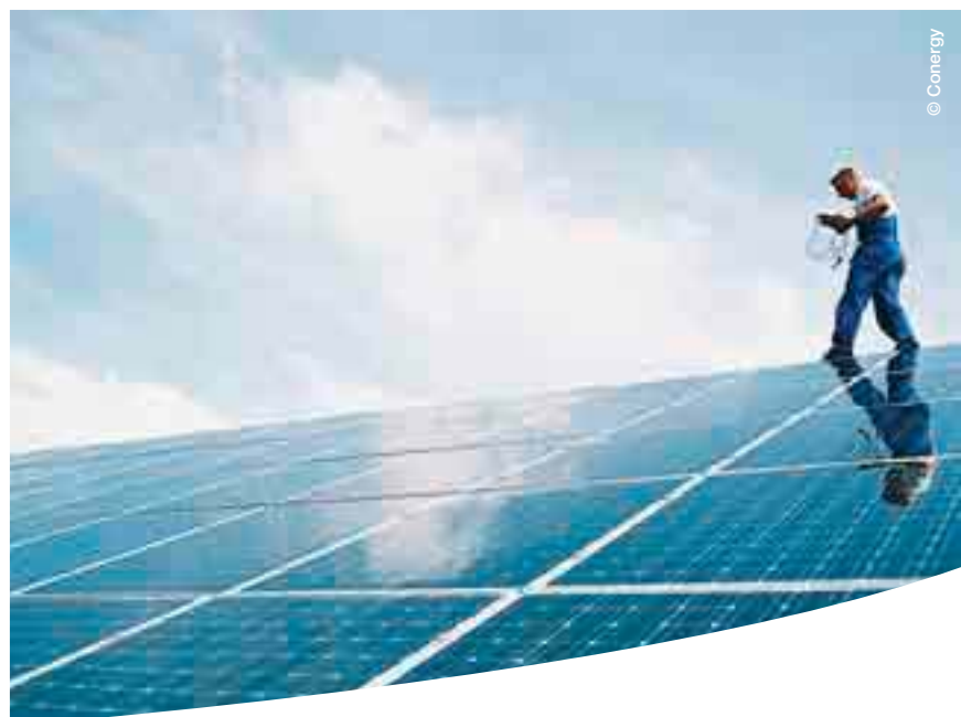
Installation of a PV system on a roof
