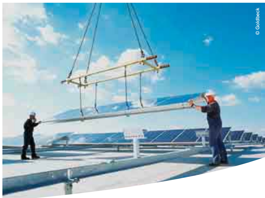
Installation of modules on a building roof
