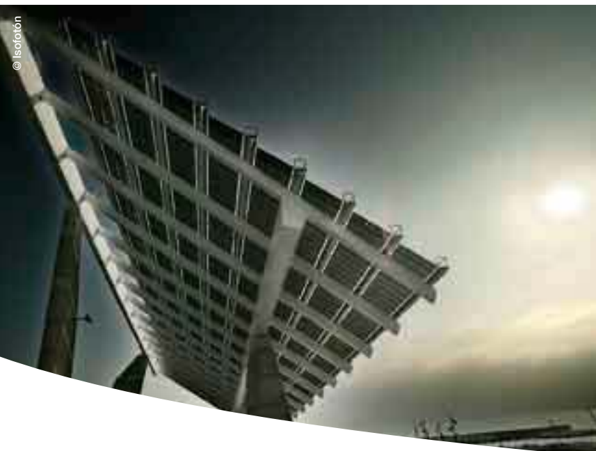
PV pergola on the Forum in Barcelona
